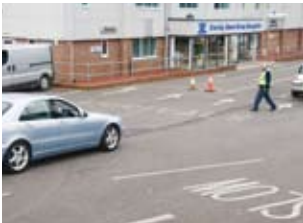
This site entrance has a segregated walkway and a marshal for directing traffic
