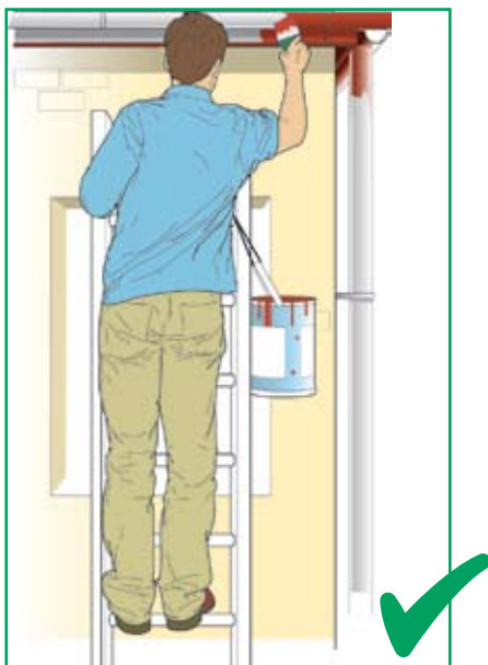
Figure 3a – This is an example of using a ladder safely by keeping three points of contact with the ladder (two feet and one hand)
