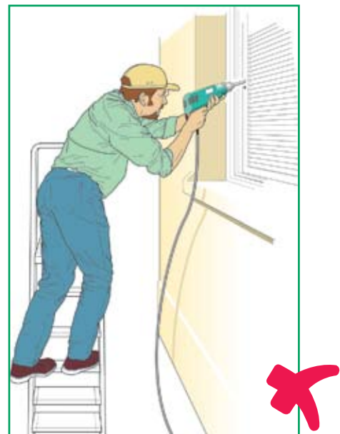
Figure 4b – This is an example of not using a stepladder safely by placing it side-on to the work
