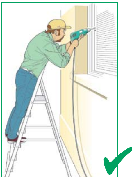
Figure 4a – This is an example of using a stepladder safely by placing it to face the work
